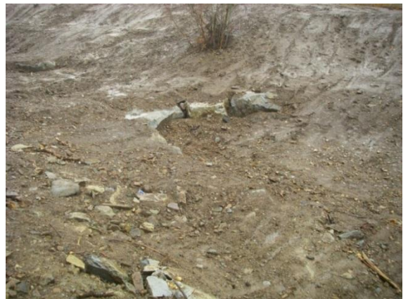
Figure 20. Restored stream channel with rock barbs (October 23, 2009).
