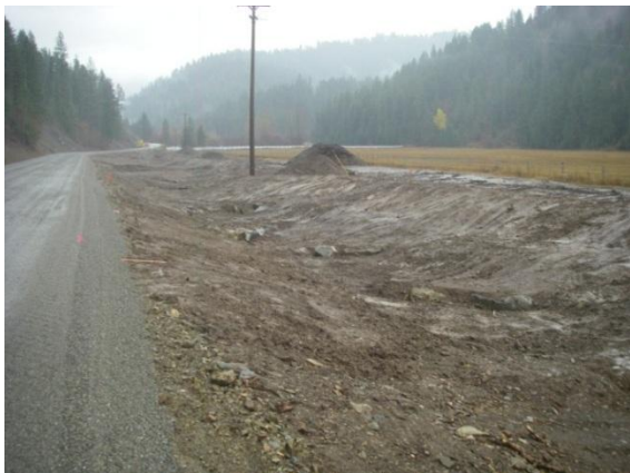
Figure 20. Restored stream channel with rock barbs (October 23, 2009).
