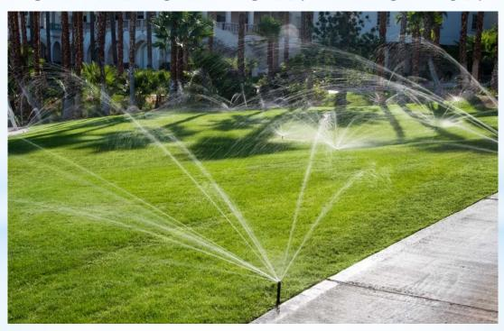
Utilize more efficient, less water consuming heads such as the MP Rotators. Use matching heads. Adjust pressures. Too much is as bad as too little.
