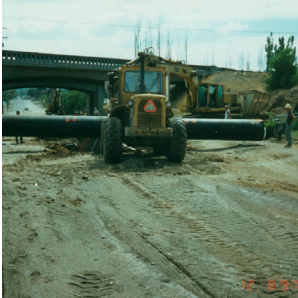
A septic tank (top) and sewer pipe installation (bottom)
